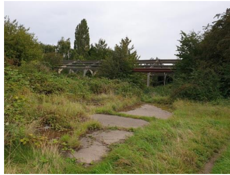
Remains of building to west of Rose Cottage
